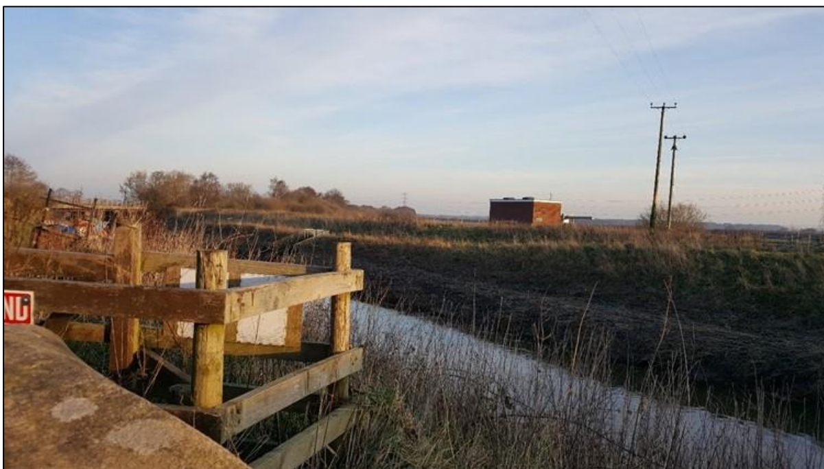
Figure 3-12 Mawdesley Pumping Station
