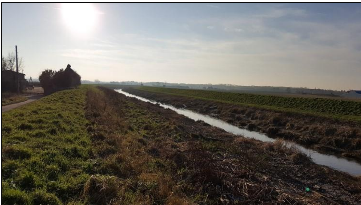
Figure 3-11 River Douglas from Meadow Lane, looking southwards
