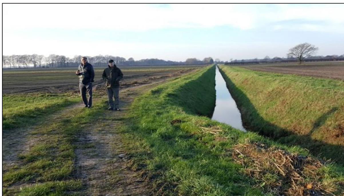
Figure 3-8 Pump Ditch (low-level), looking west
